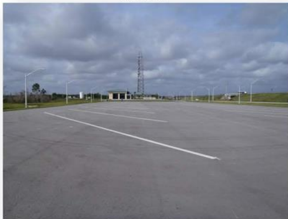
Looking west onto the new south recreational parking area and emergency response center (far end)
