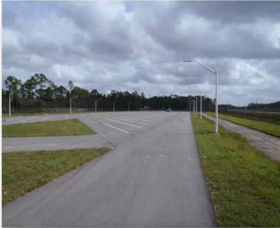
Entrance of new recreational parking area looking east; deceleration service road (west bound) is to the right.
